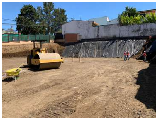
Soil works stage.
