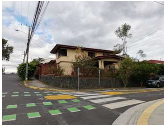
Property before the earthworks.
