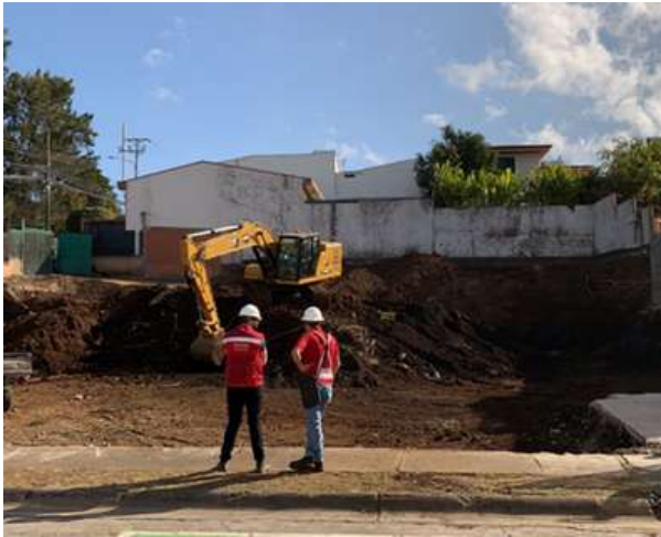
Stage 1: Earthmoving work: Base preparation for new metallic structure
