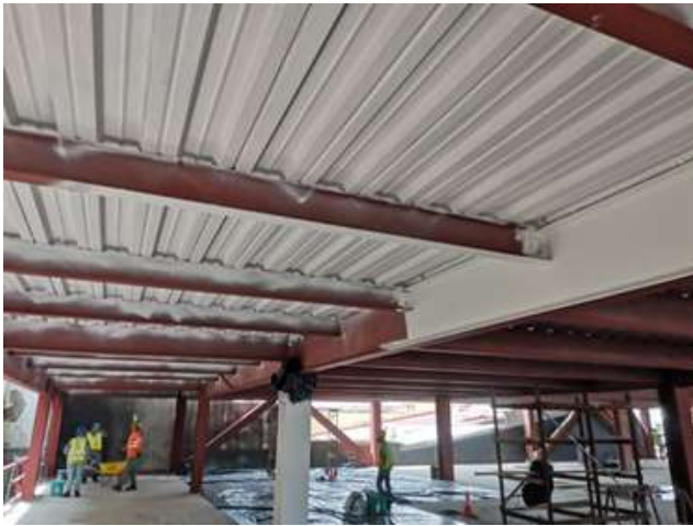
Stage 3: Installing the intumescent paint.
