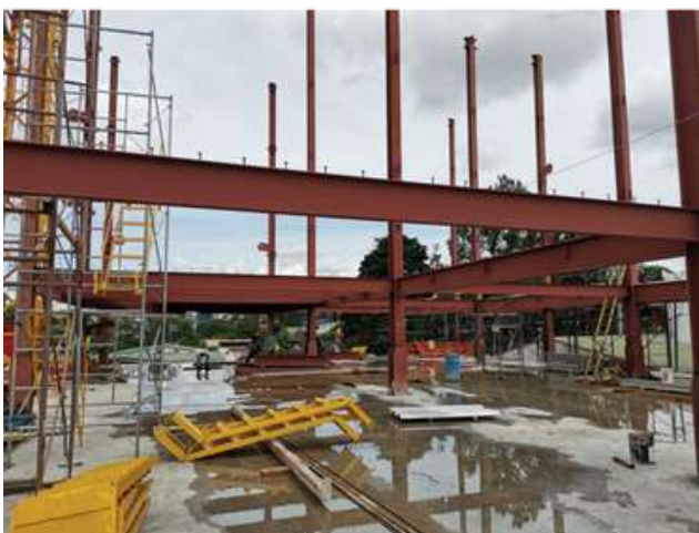
Stage 2: Foundations and metallic structure in the new building. Concrete castings
