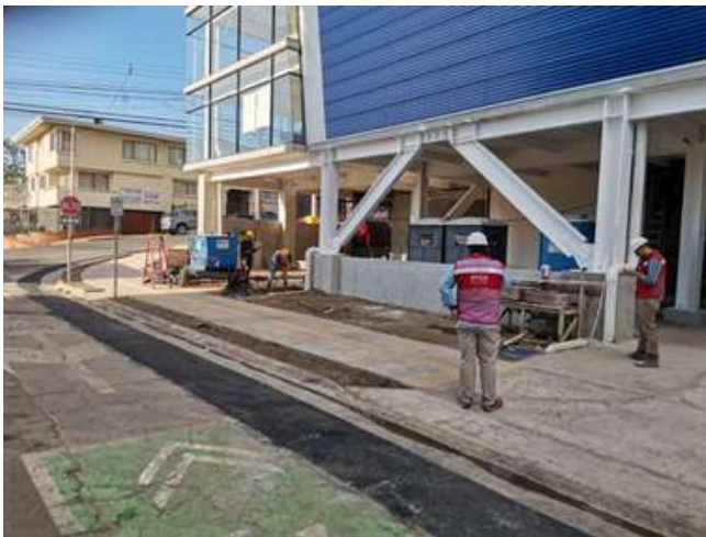
Final stage of facade details. Colored metal sheets and front windows, louvers, and administrative offices.
