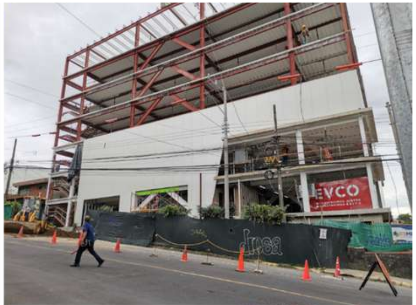
Stage 3: Installing the intumescent paint.
