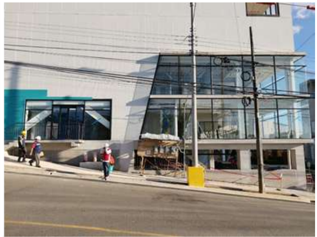
Final stage of facade details. Colored metal sheets and front windows, louvers, and administrative offices.
