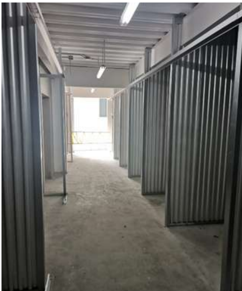
Stage 4: Installing the facade, unit partitions, and hallway system
