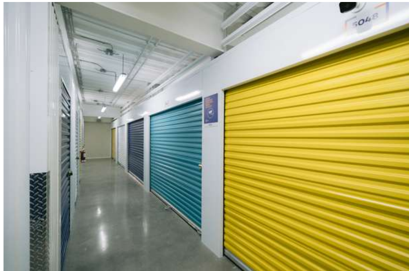
Hallway with polished concrete floor, electrical installations, and hallway system.
