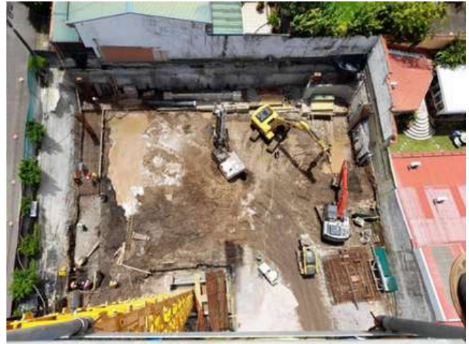
Stage 1: Earthmoving work: Base preparation for new metallic structure
