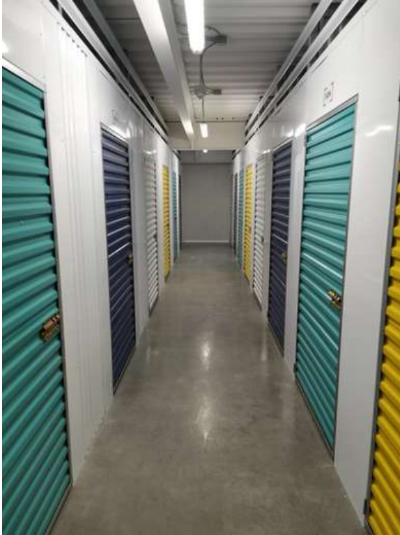
Partitions and hallway system installed.
