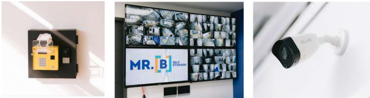
CCTV System: Includes up to 69 cameras and a set of screens where the guard, administrator, and clients can check at any time.
