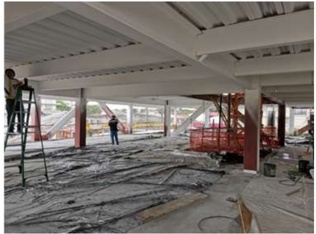
Stage 3: Installing the intumescent paint.
