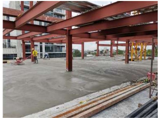
Stage 2: Foundations and metallic structure in the new building. Concrete castings
