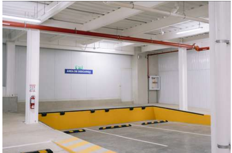
Covered unloading area
